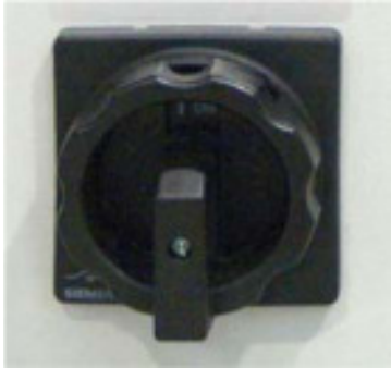
Dia. 1: Main power switch
